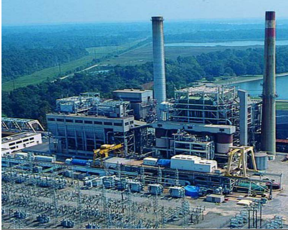
Photograph 1. Progress Energy H.F. Lee Plant.
