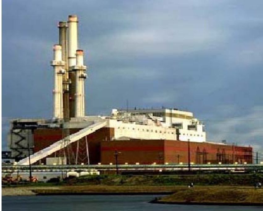
Photograph 2. Midwest Generation Will County Plant
